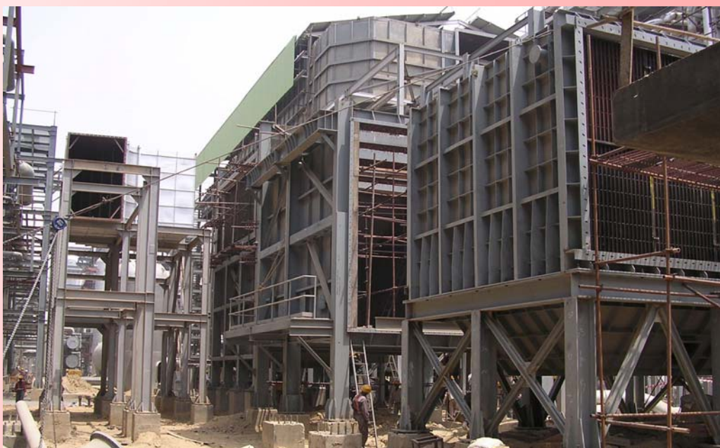
India, combustion air preheater assembling (Larsen & Toubro INDIA)
