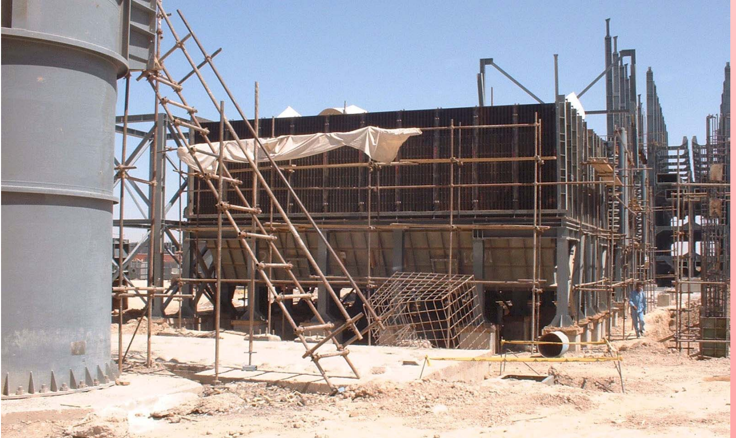
Iran, combustion air preheater assembling (SNAM PROGETTI ITALY)
