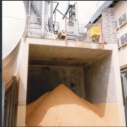
View of the separation processing on a treatment plant of timber
