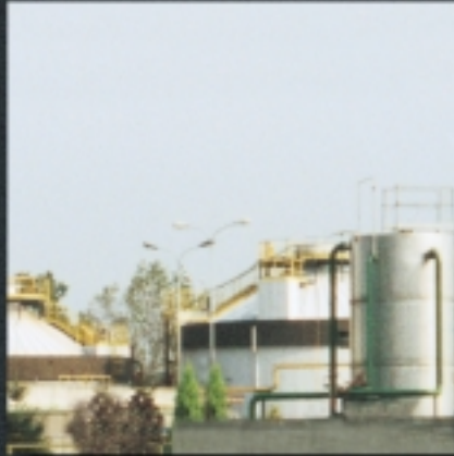
View of the purification plant
